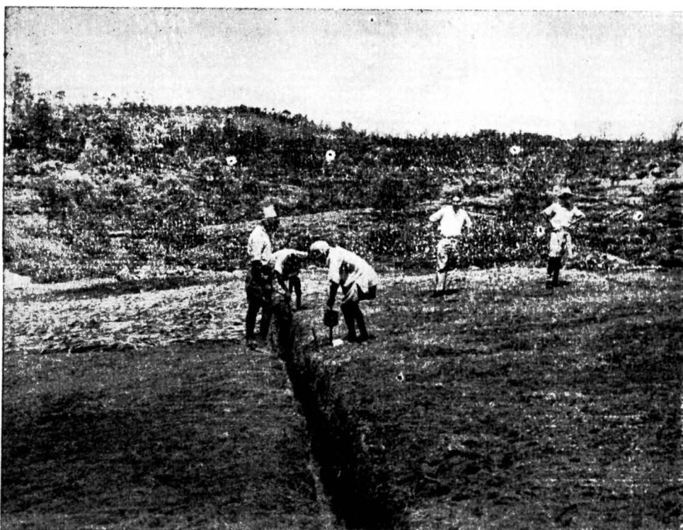
Figure 2. Fumigation with DD for control of Poria Root Disease in progress on Pundaluoya North Estate. Note fumigated area being covered with Guatemala grass loppings.
