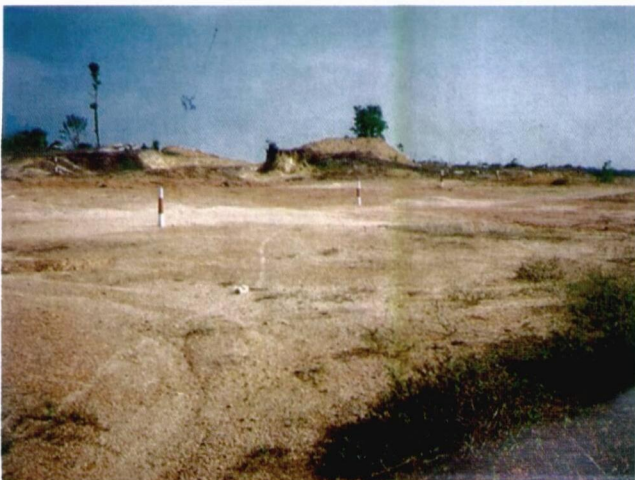
Land cleared for construction
