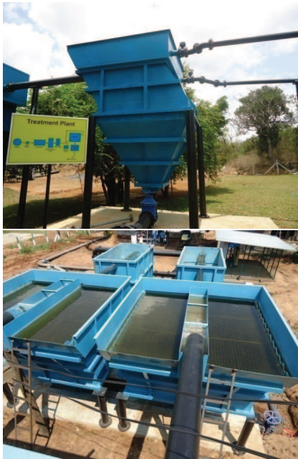
Figure 9 Tube Settlers at Thanthirimaley & Oya Maduwa by NWSDB
