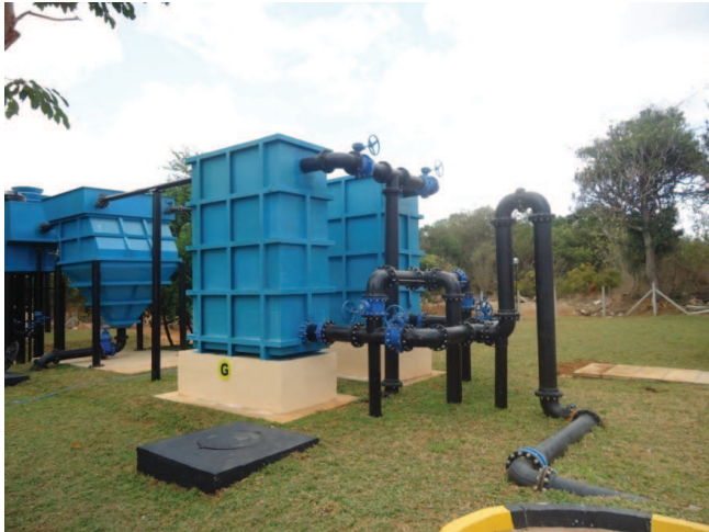
Figure 13 Domestic Slow sand filter (Bio sand filter)
