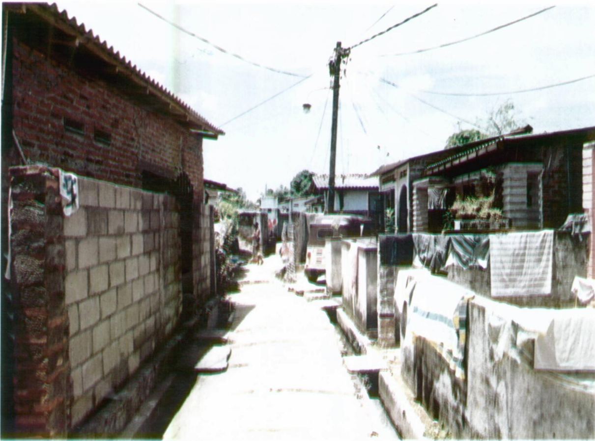
A typical street with low scale single storey housing units.
