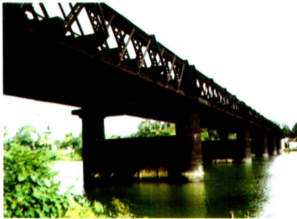
Figure 1: A view of the selected bridge
