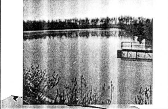
Fine particles are pumped to a settlement pond a Settling Pond
