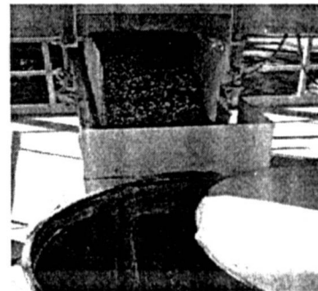
View of combined stone being fed into Vertical Shaft Impact Crusher
