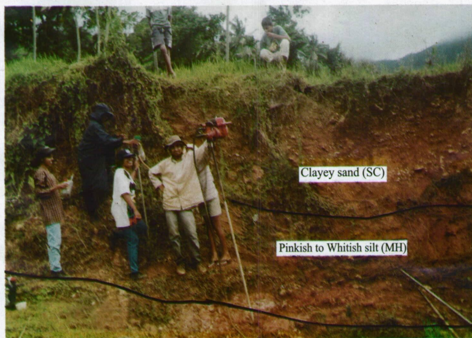
Fig. 4 Weathering Profile at the head scarp of the slope failure.
