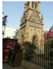
Figure 12: Lack of maintenance and care
