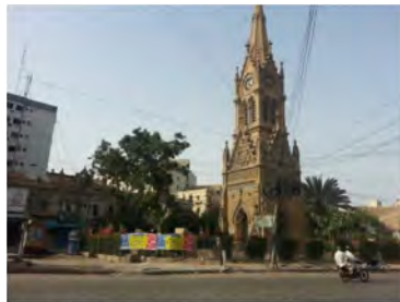
Figure 9: Electrical lines around the tower
