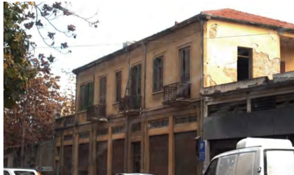
Figure 10: Façades on Paphos Street before restoration, walled Nicosia
