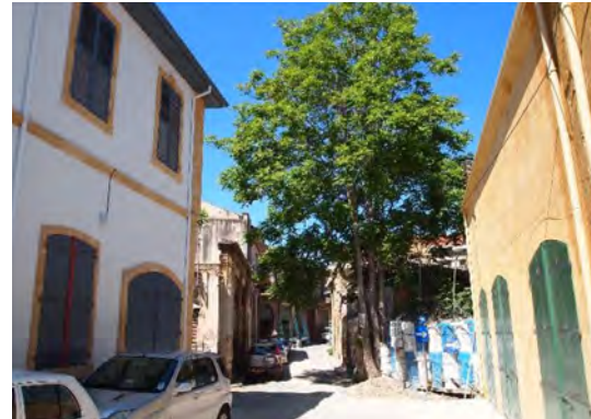
Figure 5: Restored facades at Dionisou street Source: Nicosia Master Plan Office (2014b)
