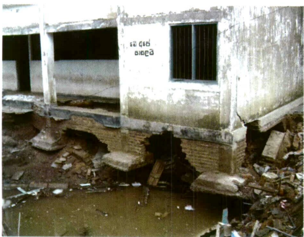
Figure 10: Under-scouring of foundation at a corner of a school building from tsunami waves
