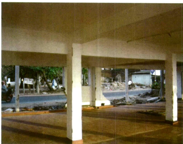
Figure 8: A structure of a building survived with minimum damage. Only the infill masonry panels have collapsed from tsunami waves
