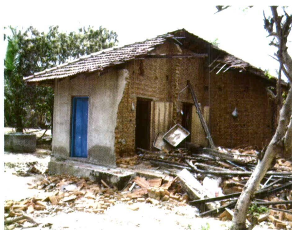
Figure 7: Partially collapsed brickwork structures due to tsunami tidal waves in Sri Lanka
