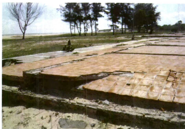
Figure 9: Failure of a masonry low rise building in Yala-Safari Beach Hotel, Yala, due to tsunami waves
