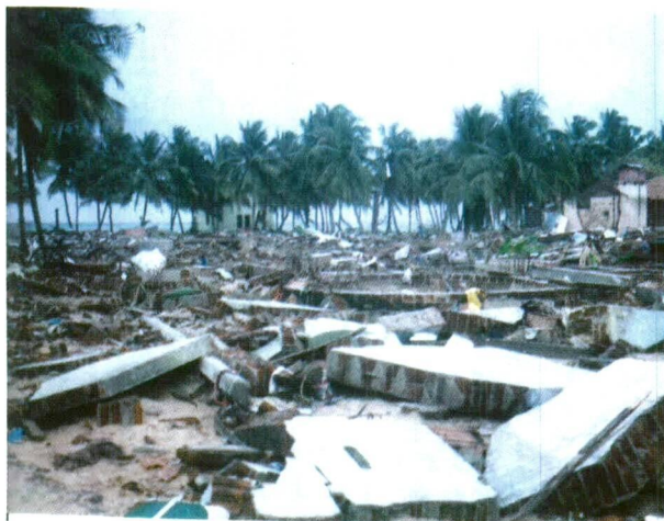
Figure 6: Completely collapsed brickwork structures due to tsunami tidal waves in Kalmunei
