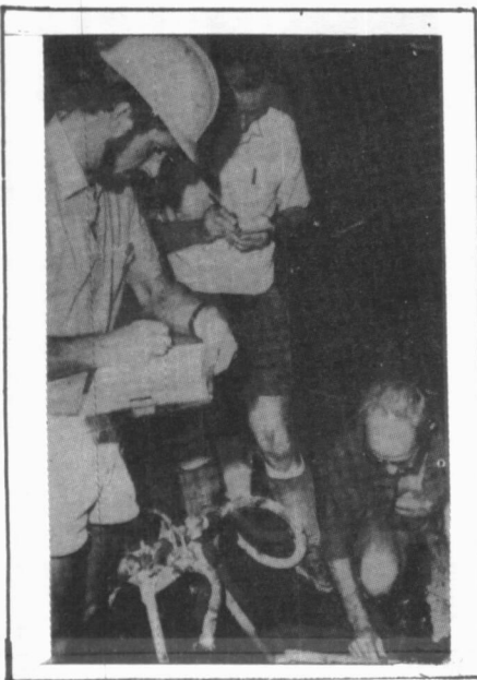
Expatriate personnel working in a project site
