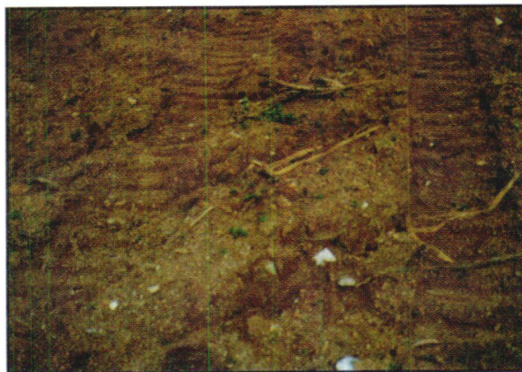
Plate 2. Soil is compacted due to heavy machine movement over the soil
