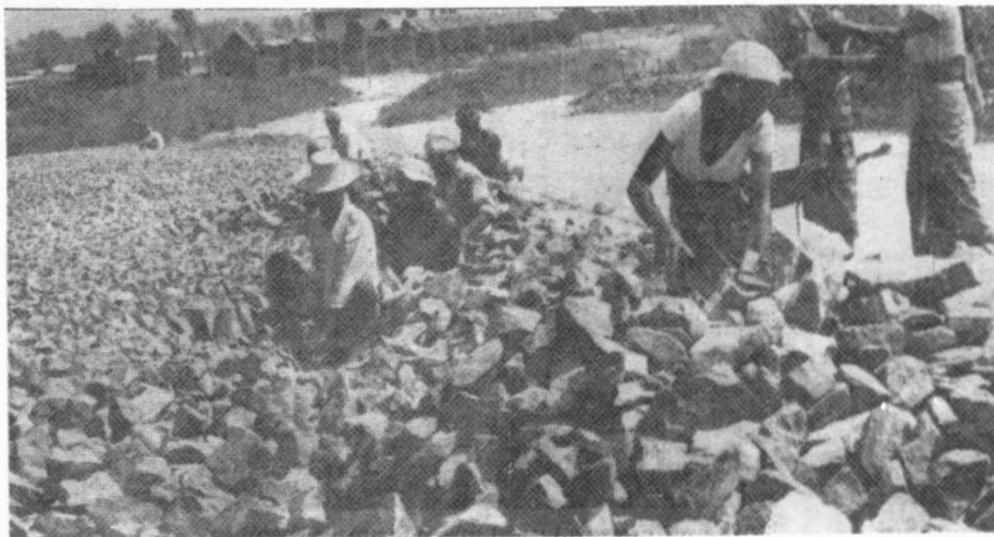
Road construction with Local Labour in System "C"
