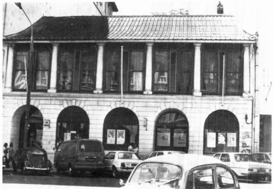
Fig. 4. Air Lanka office, Prince Street. A late eighteenth or early nineteenth-century building in which the arcade and colonnade were probably open originally.
