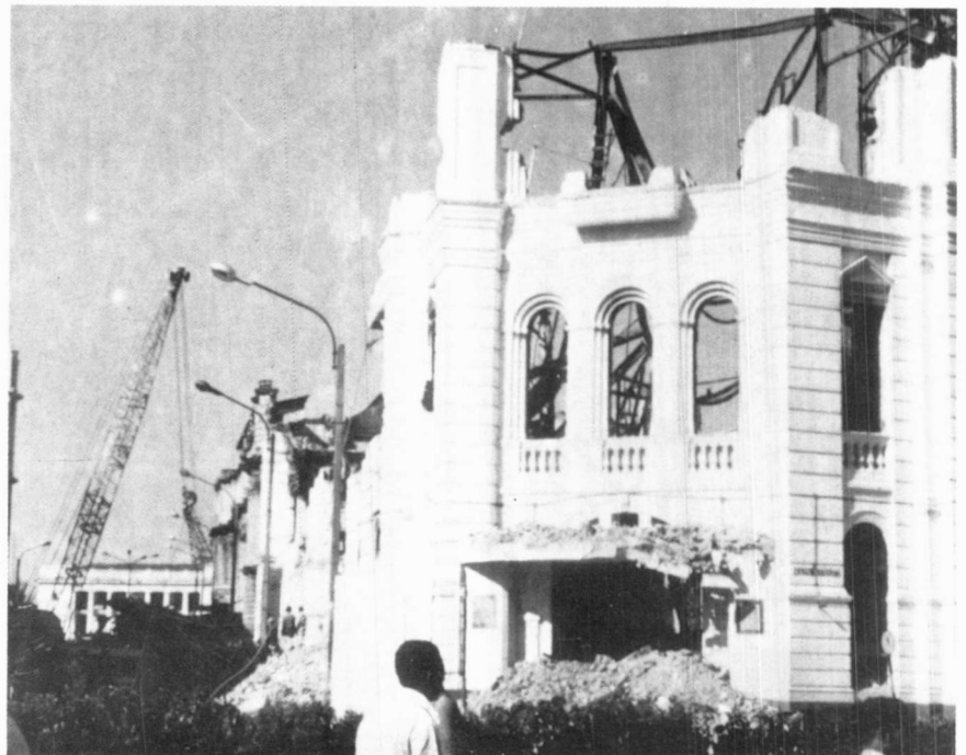
Fig. 1. The demolition of the fire-damaged Grindlays Bank, York Street.
