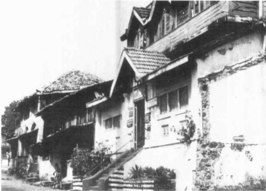
Fig. 13. Buildings at the corner of Mibindu Mawatha and St. Sebastian Hill.
