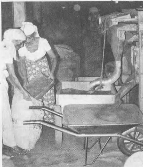
Plate 10 Screening of graphite flakes using vibrating screen. Kahatagaha Kolongaha mine
