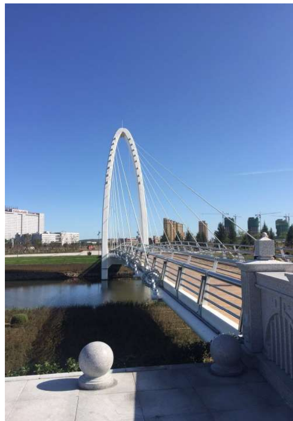
Figure 1: Picture of the pedestrian bridge
