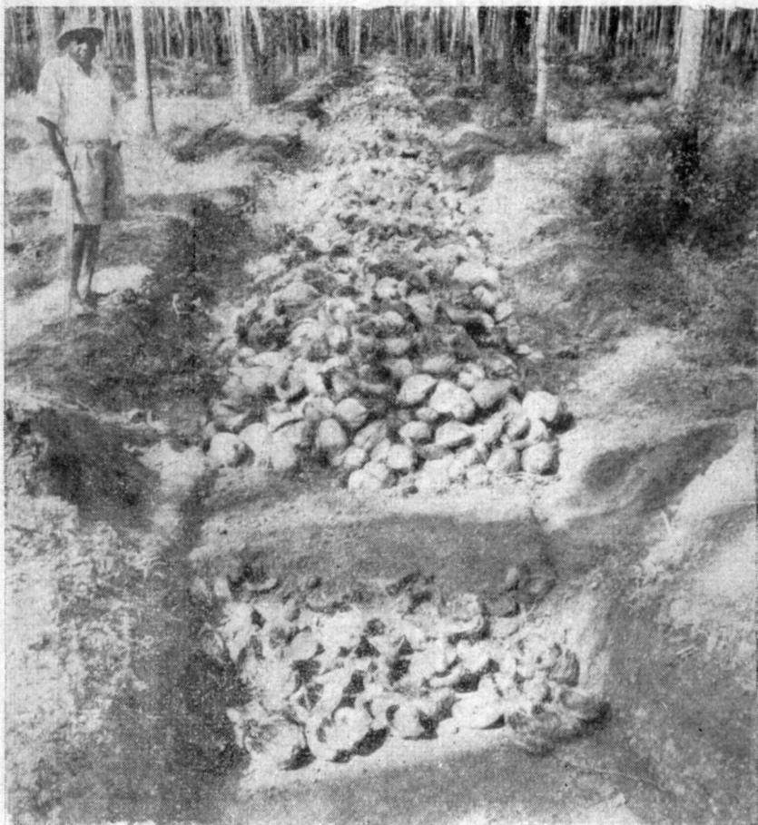
Husk Bund Husk Bund Under Construction
