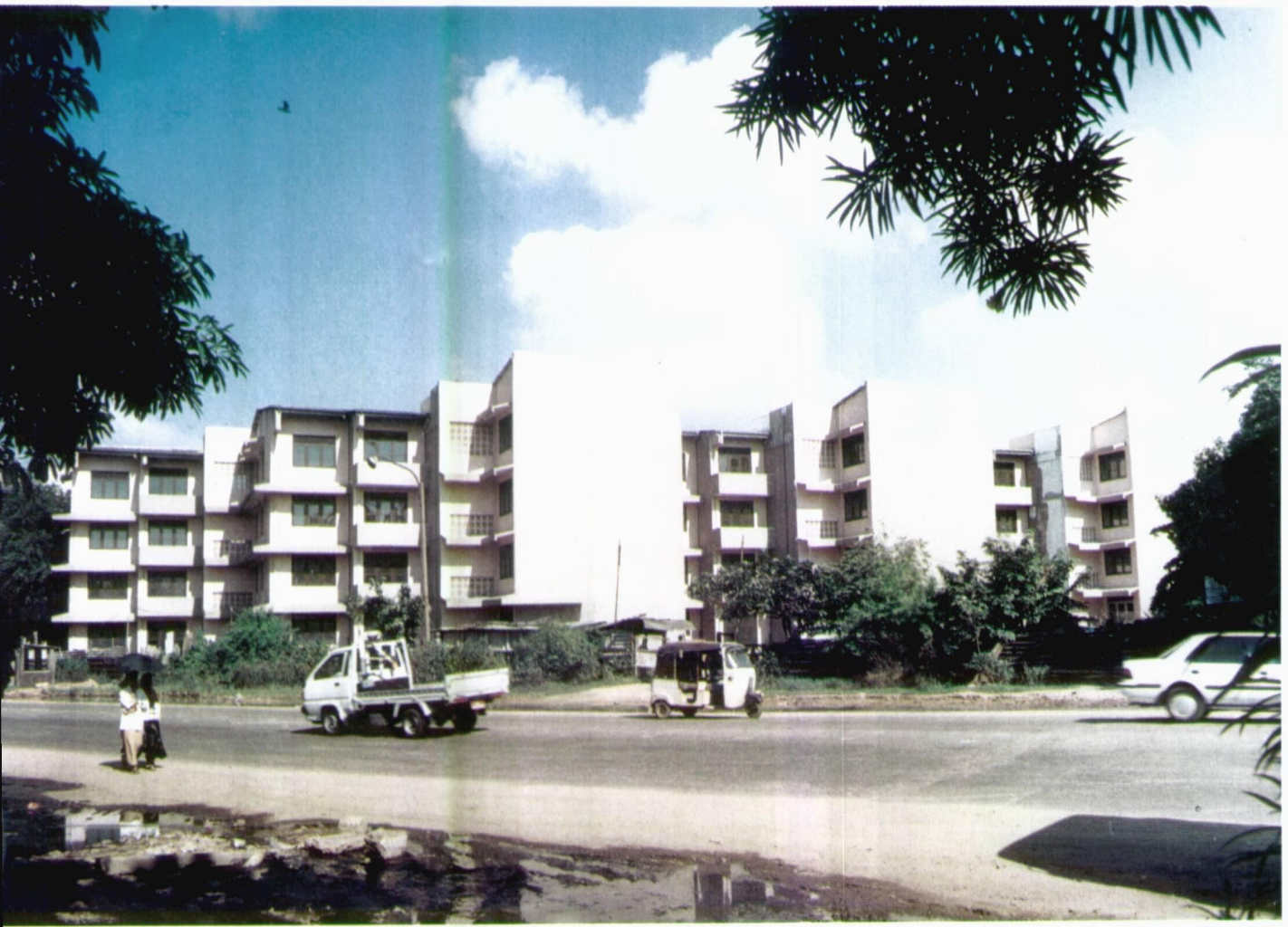
Maligawatta Housing Scheme
