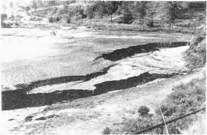
Figure 4.6: Accumulation of silt on the bed of Norton Bridge Reservoir after 30 years, the result of soil erosion of the surrounding slopes.
