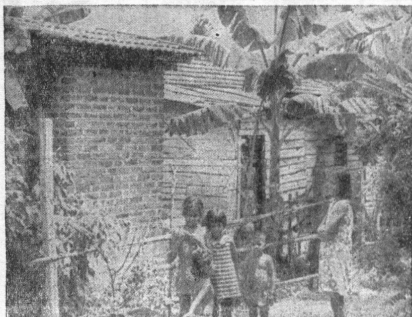
One recognised system whereby populations with irregular or low incomes could improve their housing by their own efforts is through self-help schemes.
