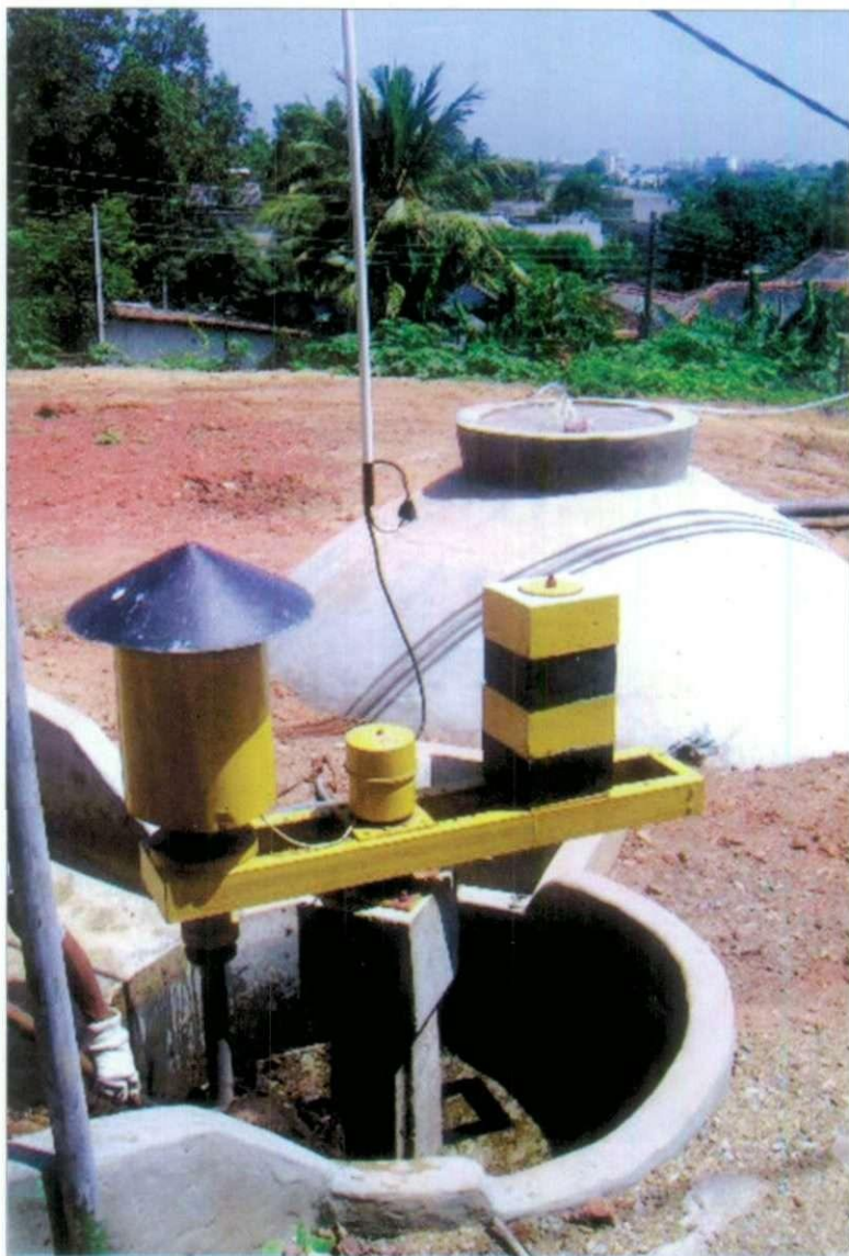
Bio gas plant at Dehiwala Zoo
