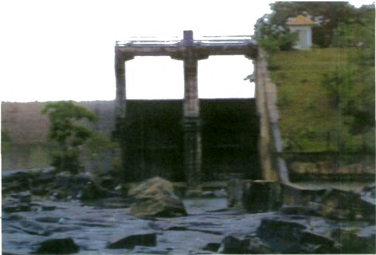
Plate 7: Spillway at Kalavava
