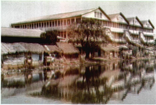
Prior to upgrading.
