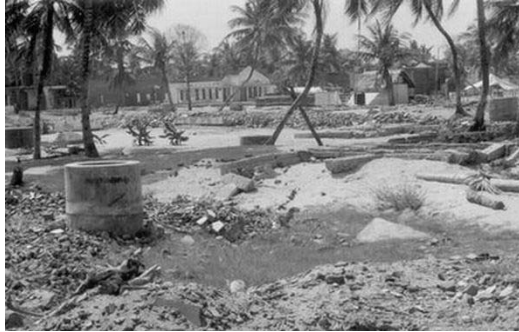
Figure 6: Almost total destruction of a coastal village. Wave heights were over 11 m here. Note cylindrical water wells. Location: Maruthamunai (East Coast, Amparai district).
