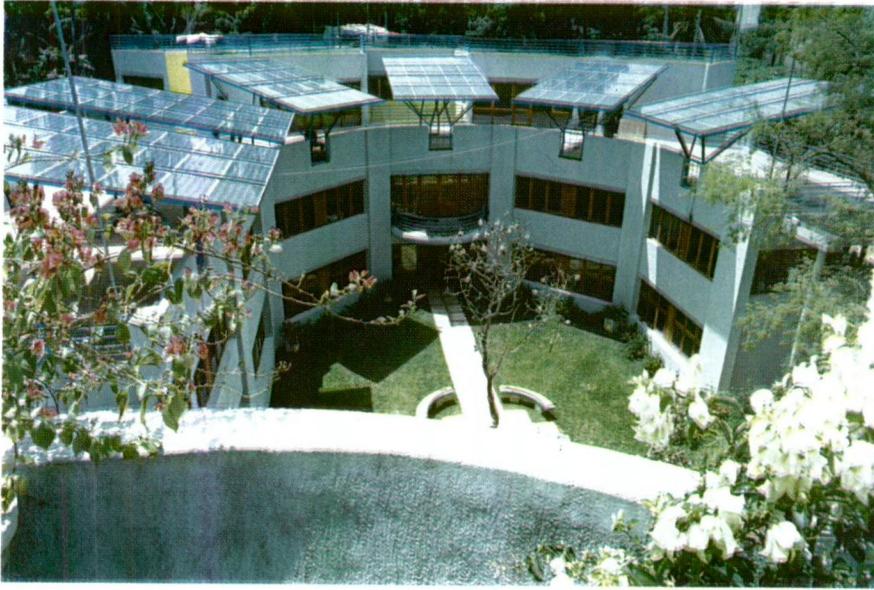
Solar panels on second floor slab when completed, the space underneath the panels will be used as meeting places for the various departments.
