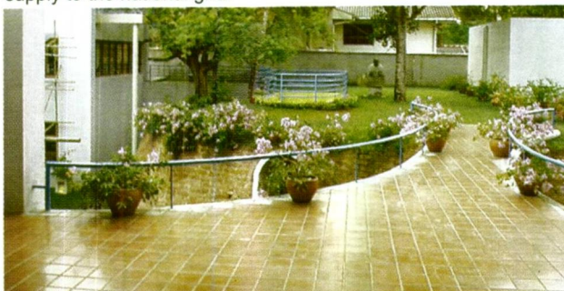
Bridge leading to birms created over air conditioned areas for insulation of the areas against heat gain
