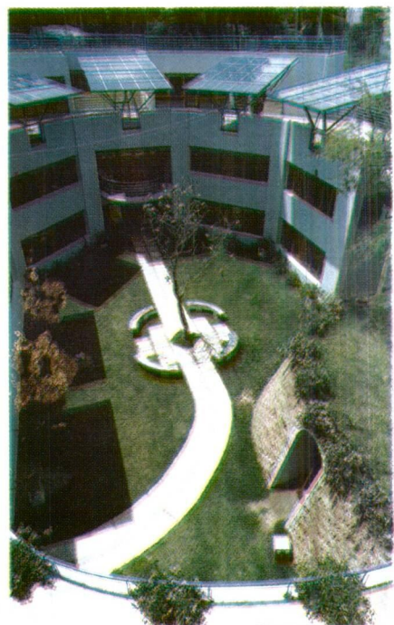
Solar panel above second floor
