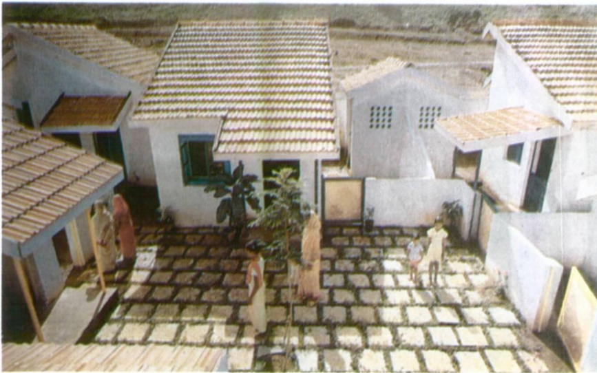
Belapur – A courtyard.
