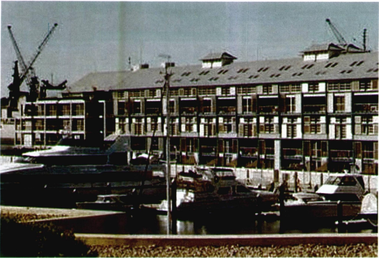
Walsh Bay apartments Finger Wharf
