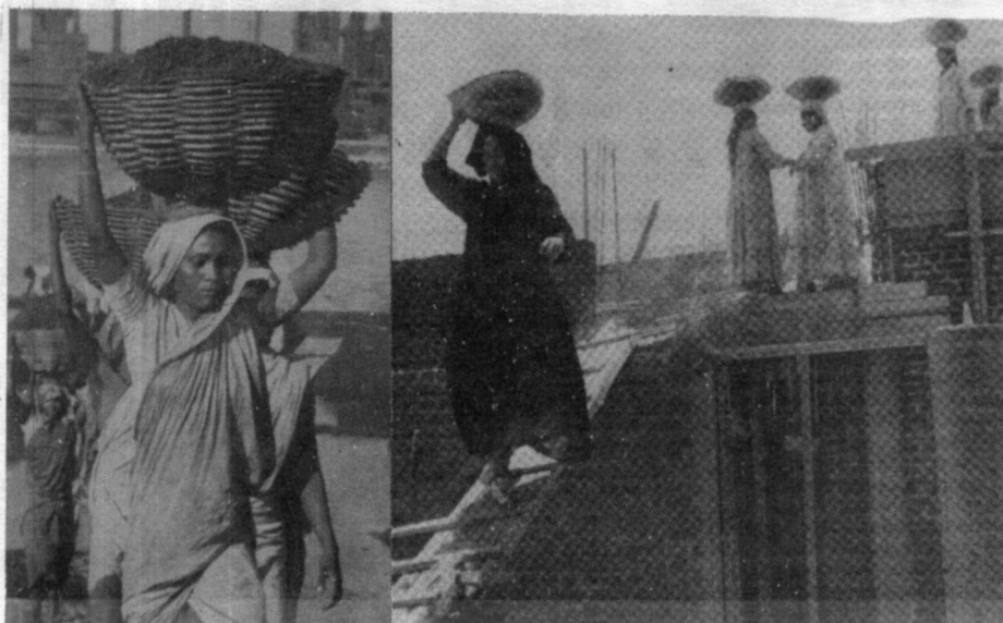
The contradiction between the image of "frailty" and "docility" of women aspiring for jobs and those who have to engage in hard manual labour is best seen at construction sites the world over, as these pictures of 'Women at Work' in Egypt and Delhi would illustrate.
