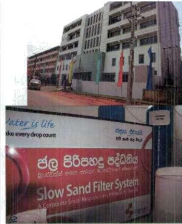
A'Pura Kidney Hospital – Slow Sand Filter Project
