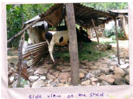
One of the cattle sheds before project implementation
