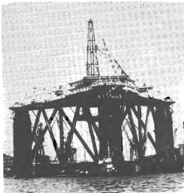
Fig. XVI A giant fixed oil-drilling platform. This 3000 ton platform can drill up to 2500 metres deep.
