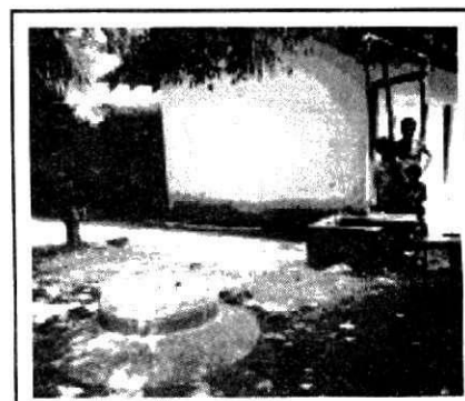
Figure 5: Partially underground tank
